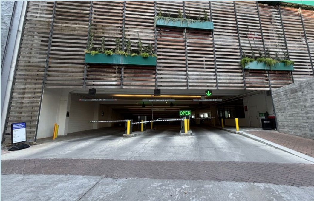
Parking garage entrance on Simond Avenue
