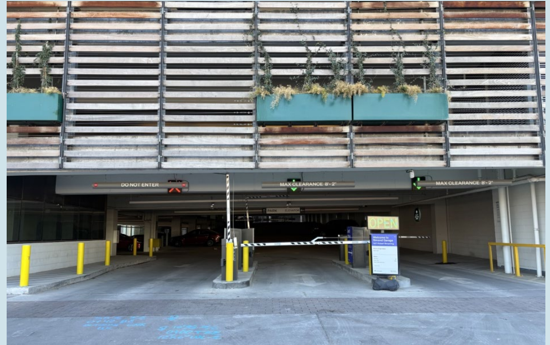
Parking garage entrance on Robert Browning Street
